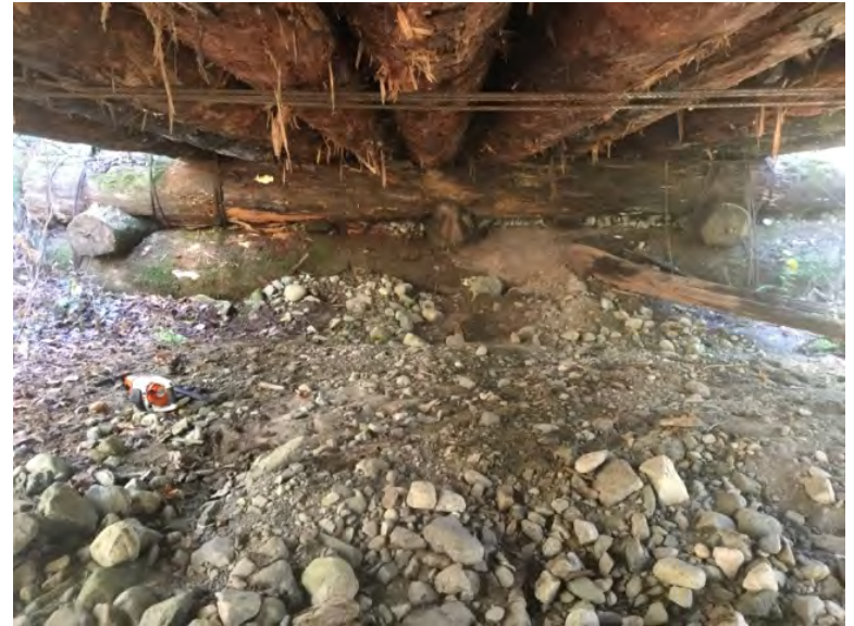
Left Bank Abutment when facing downstream
