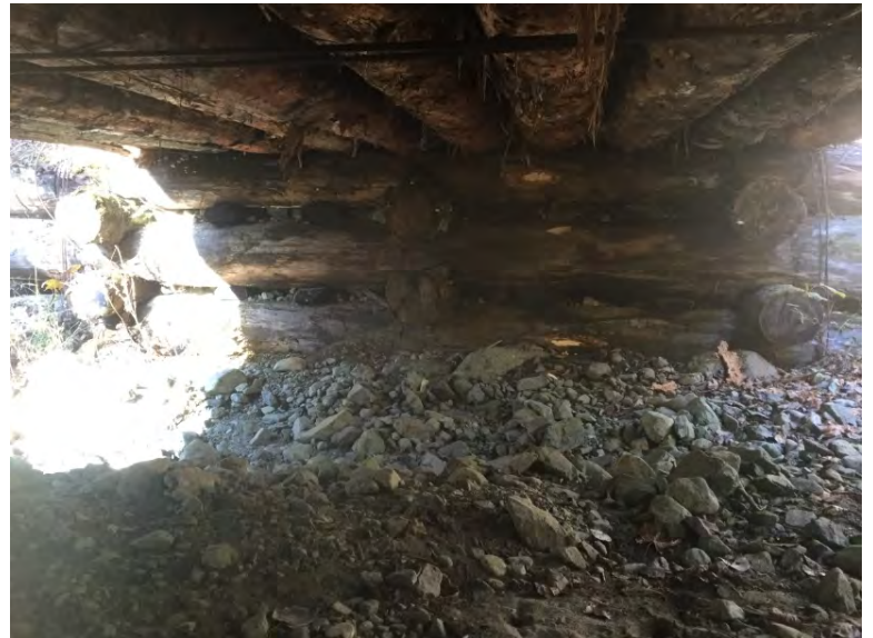
Right Bank Abutment when facing downstream
